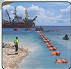
Cebu-Negros-Panay 230kV Backbone Energized - March 2024
