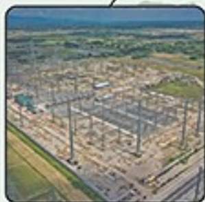
Mariveles-Hermosa-San Jose 500kV Transmission Line Energized - June 2024
